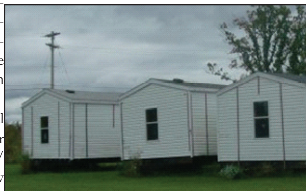
Replacement FEMA Manufactured Homes
